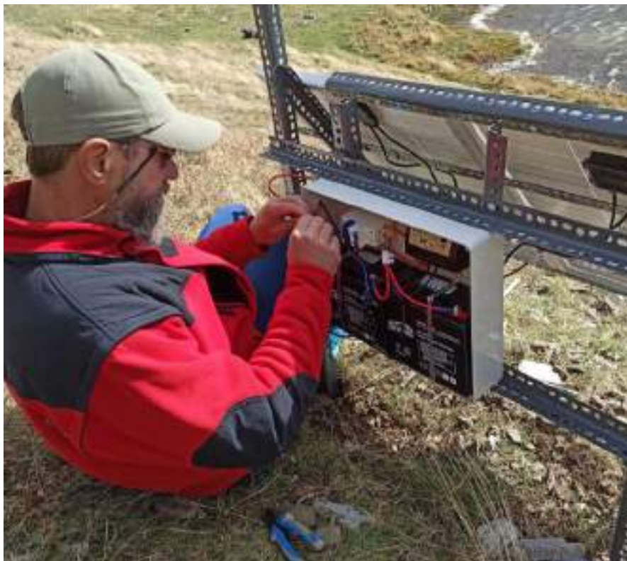
Figure 19. Connecting the solar panels with the batteries.
